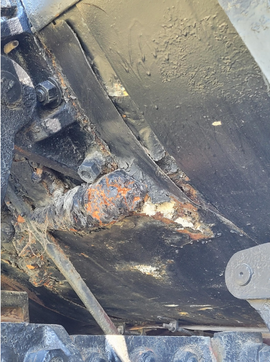
Rust and Jagged Edges
