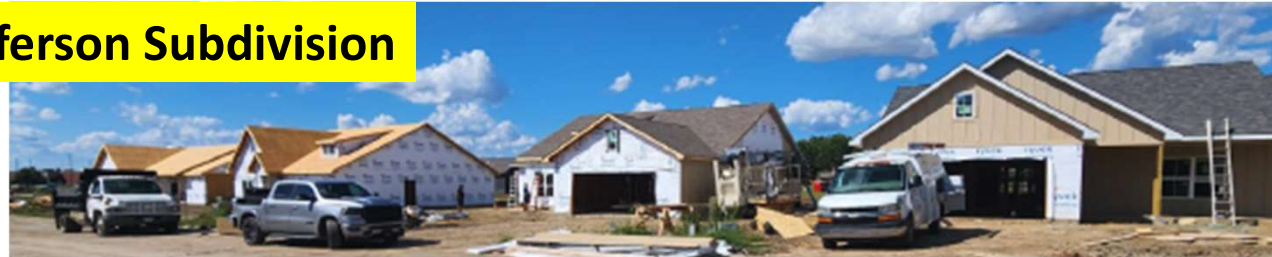
Independence Housing Authority Eight Homes Under Construction
