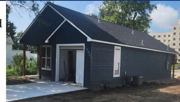
Diamond Properties LLC Two Infill Homes Completed
