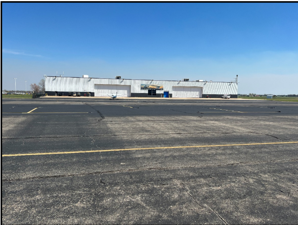
Existing Condition of North Apron
