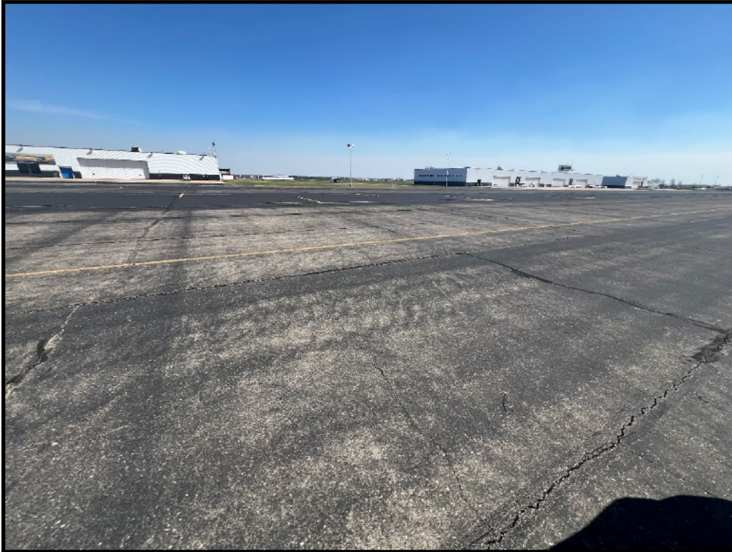
Existing Condition of North Apron
