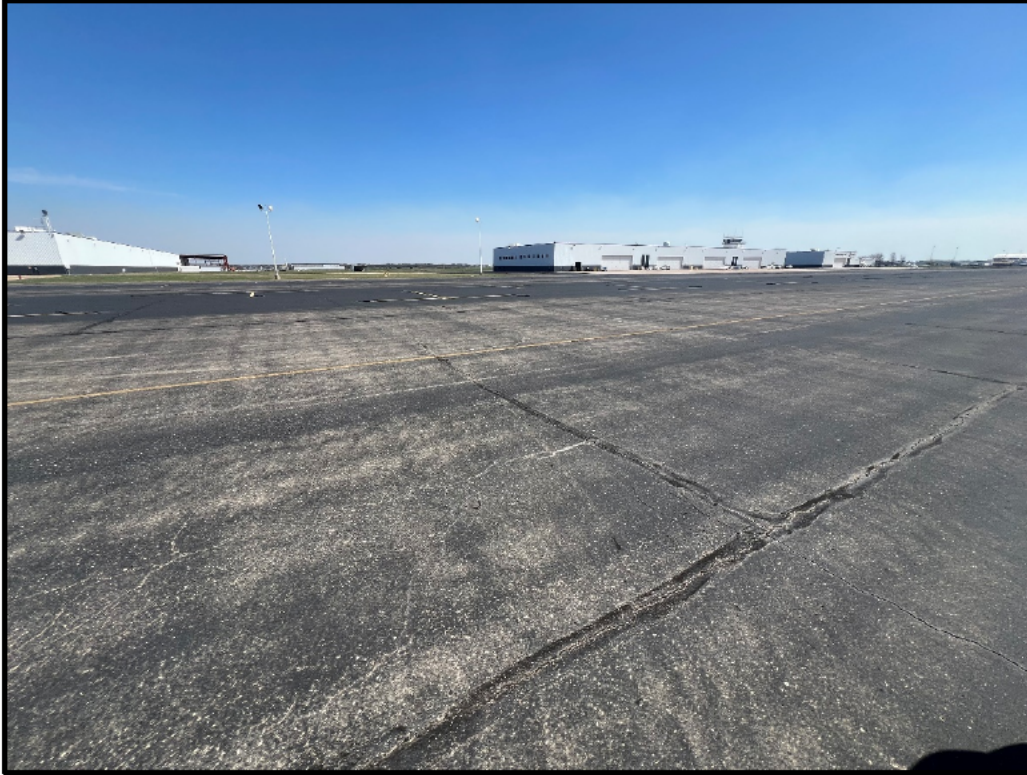
Existing Condition of North Apron
