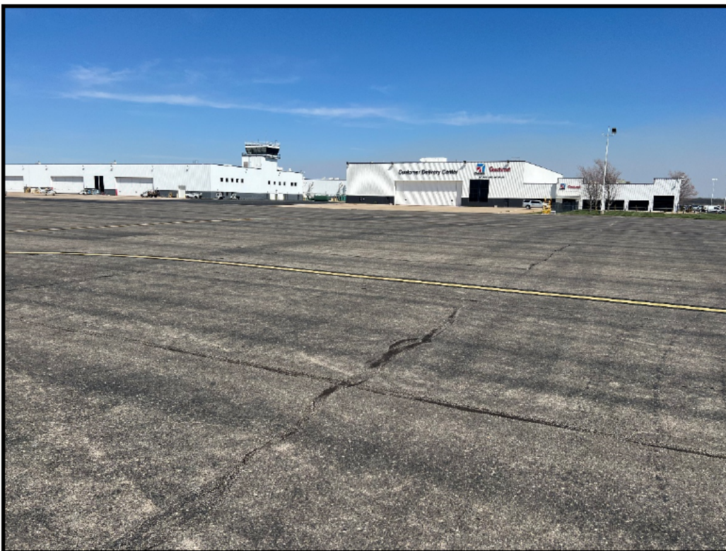
Existing Condition of North Apron
