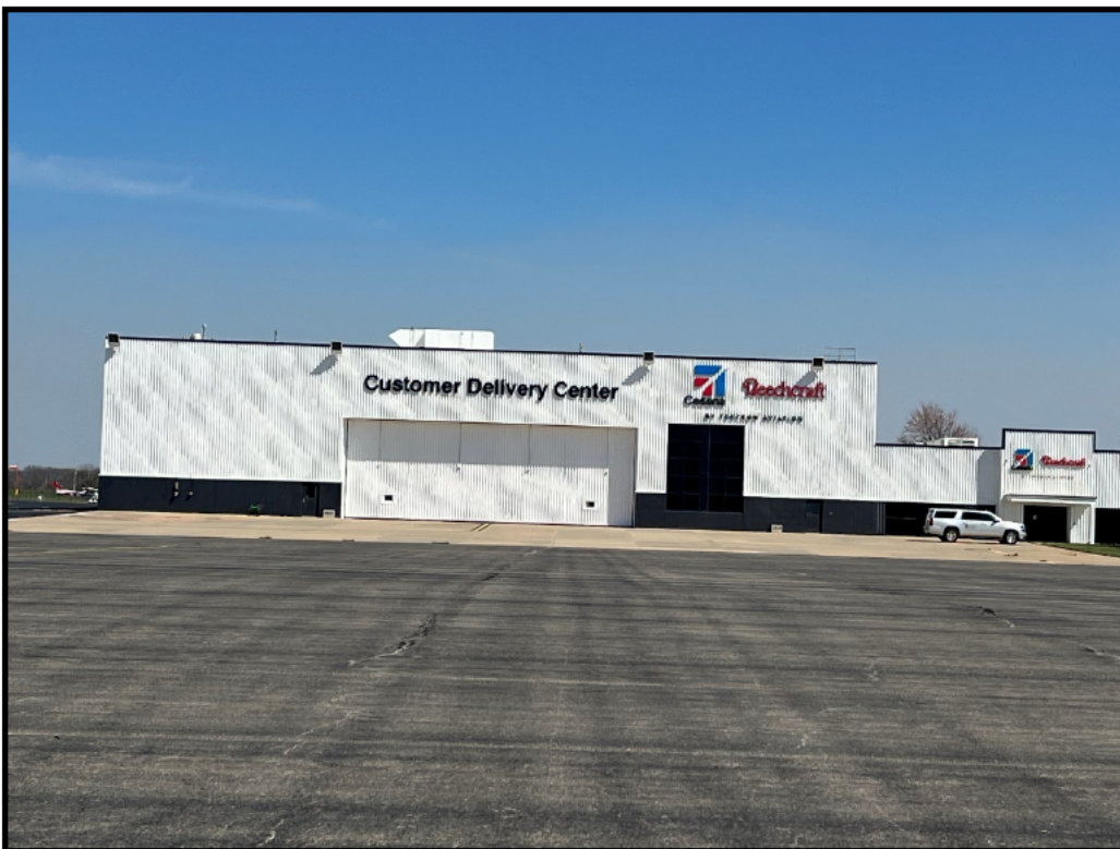
Existing Condition of North Apron
