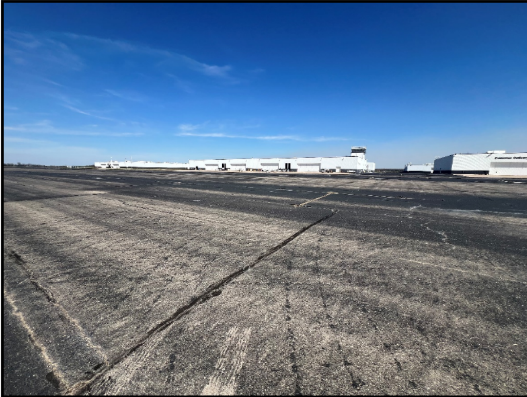
Existing Condition of North Apron
