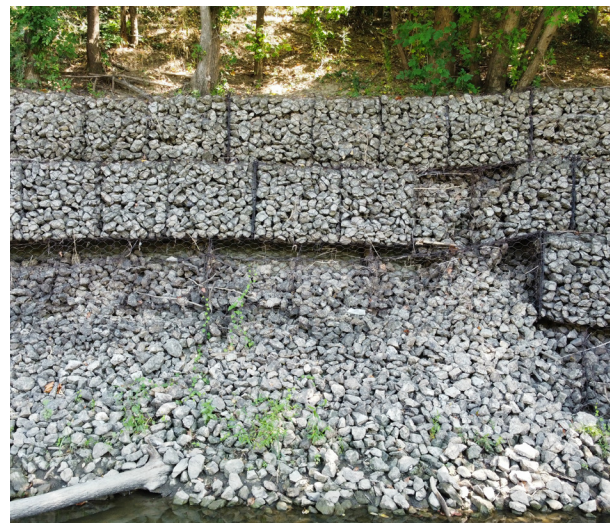
Figure 3. Gabion failure
