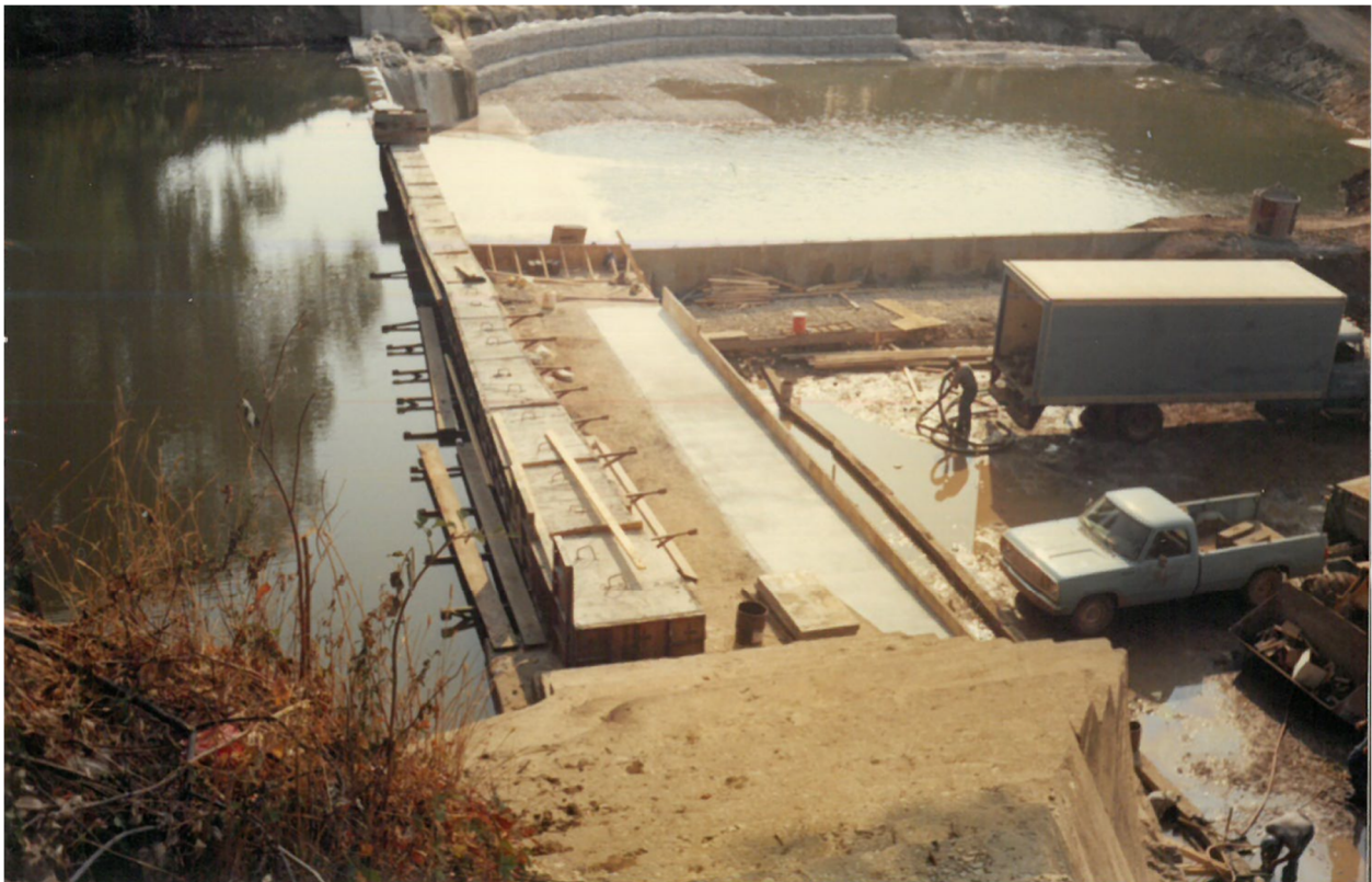
FIGURE 8 - APRON EXTENSION AND REPAIR COMPLETED, SEPTEMBER 14, 1988
