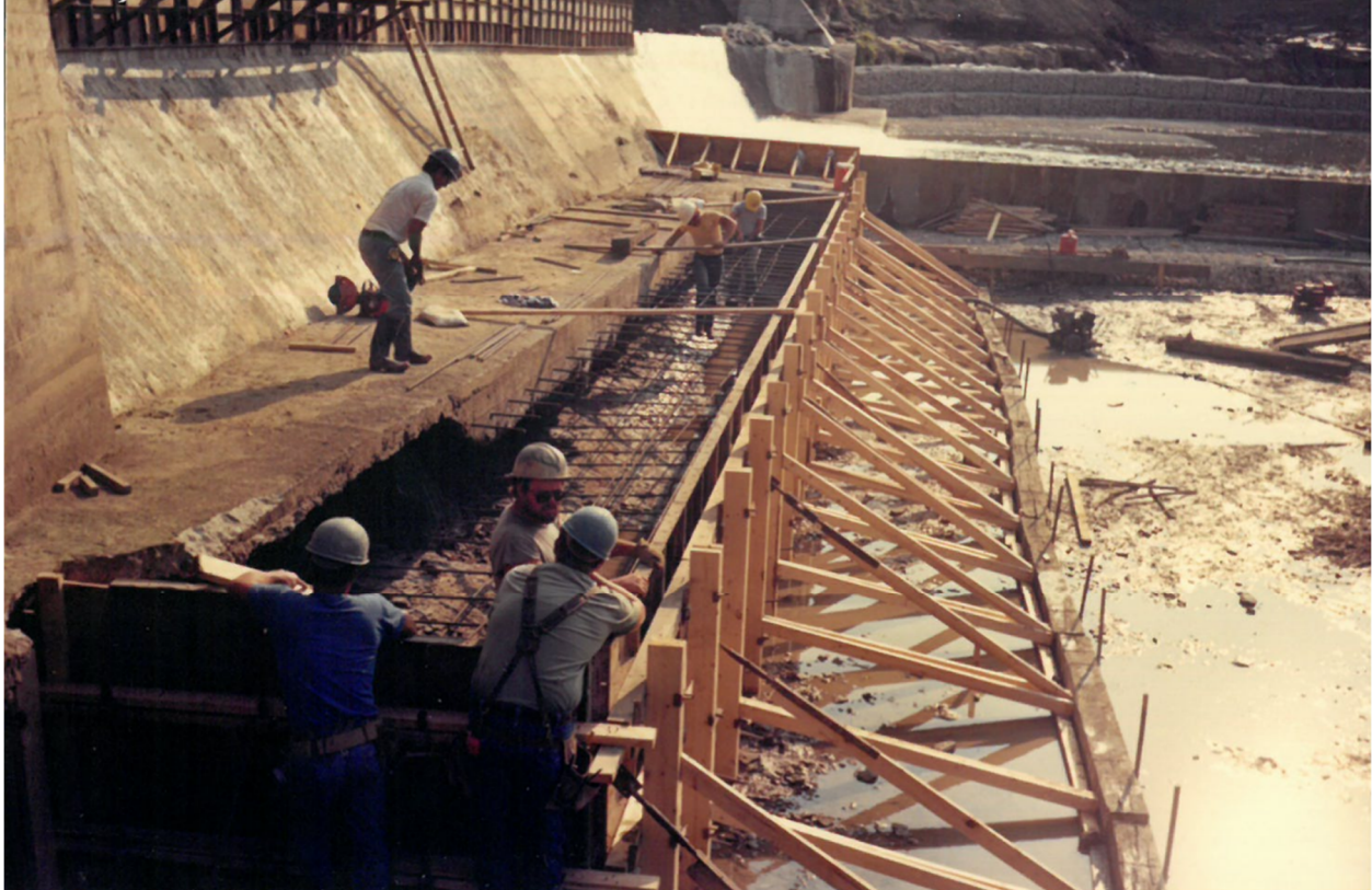
FIGURE 7 - SCOUR REPAIR AND APRON EXTENSION UNDERWAY, SEPTEMBER 13, 1988
