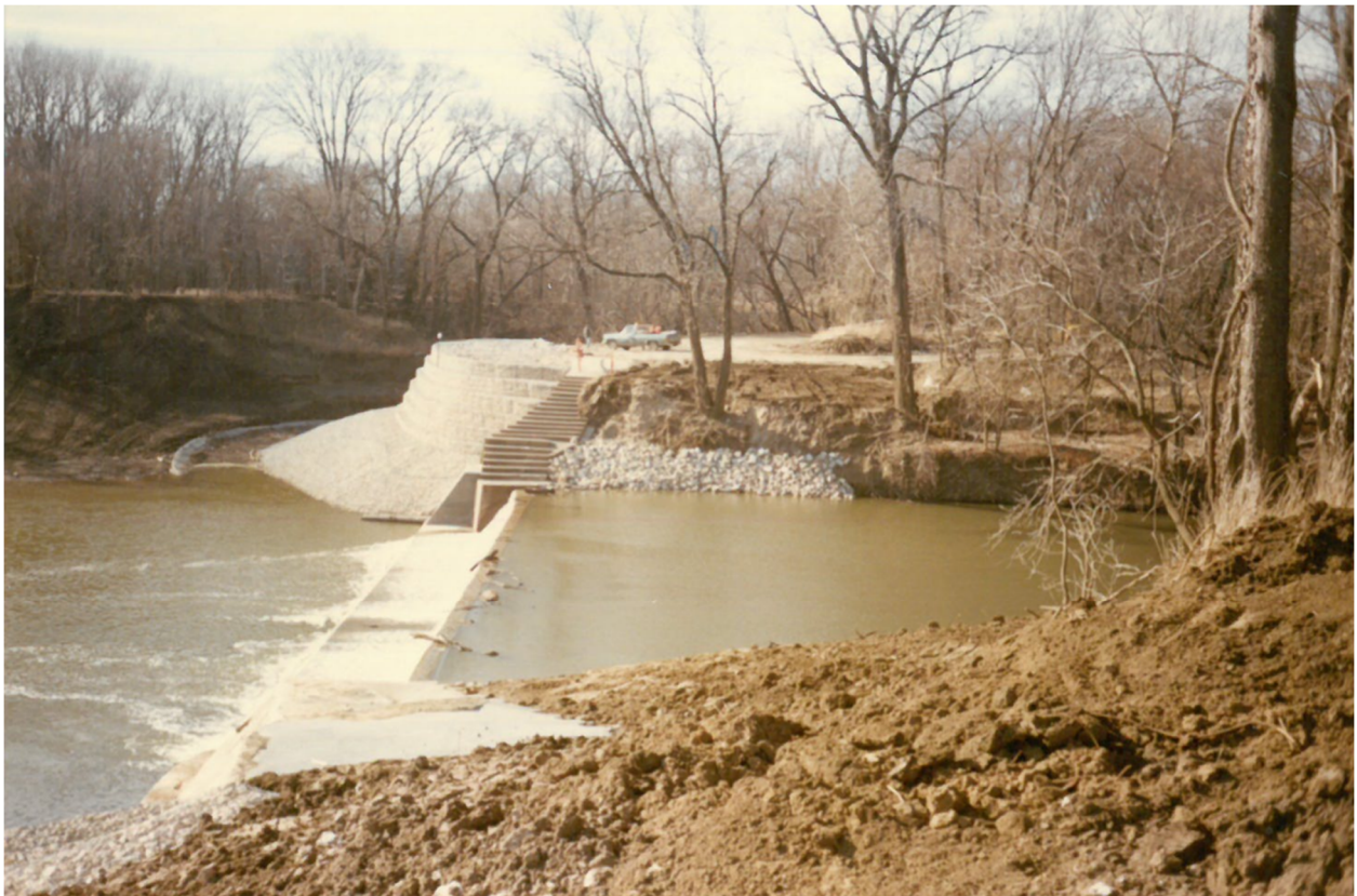
FIGURE 10 - UPSTREAM RIPRAP PLACED, PROJECT COMPLETION, JANUARY 5, 1989
