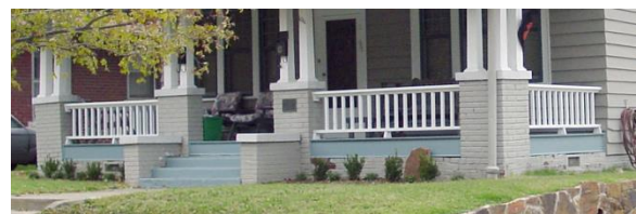
Traditional design with railing lower than piers.
