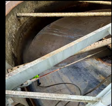
Shut down clarifier for cleaning.
