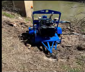
6" Pump used to pump out the mud.
