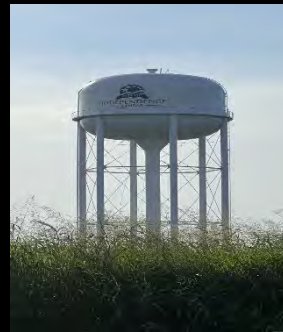
Water Tower cleaned & painted.
