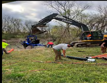
Setting the pump for the dive team cleaning the low service.
