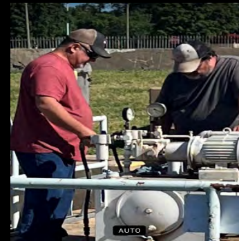
Installing new hydraulic pump.
