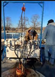
Installed new Turbine Drive Motor on the clarifier.
