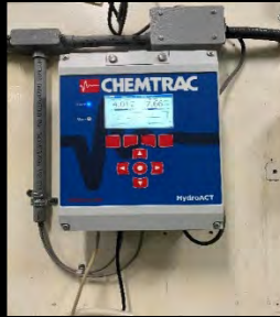
Installed new finished water Chlorine analyzer.
