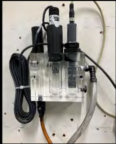
Installed new finished water Chlorine analyzer.
