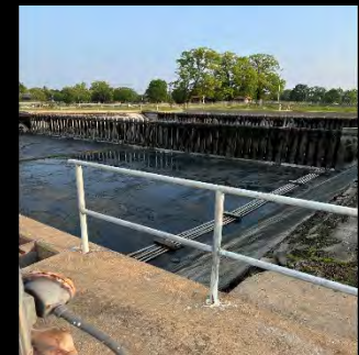
Repairing broken shafts.
