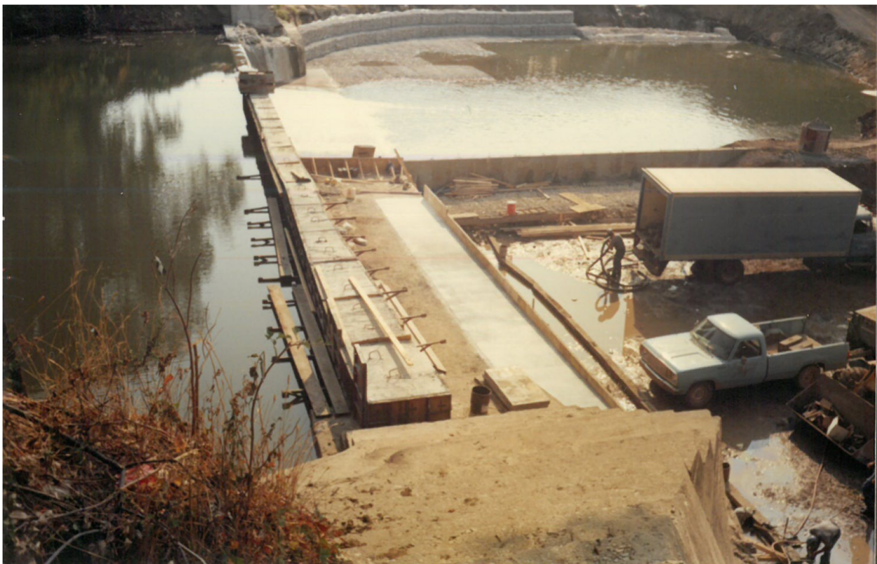
FIGURE 8 - APRON EXTENSION AND REPAIR COMPLETED, SEPTEMBER 14, 1988
