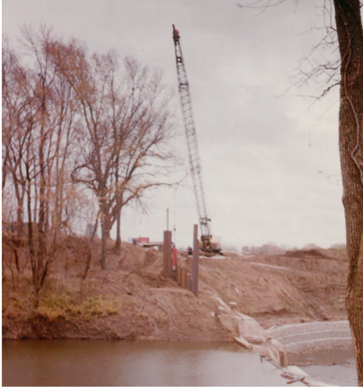
FIGURE 9 - STEEL SHEET PILE DRIVEN UPSTREAM OF EAST ABBUTMENT, NOVEMBER 2, 1988
