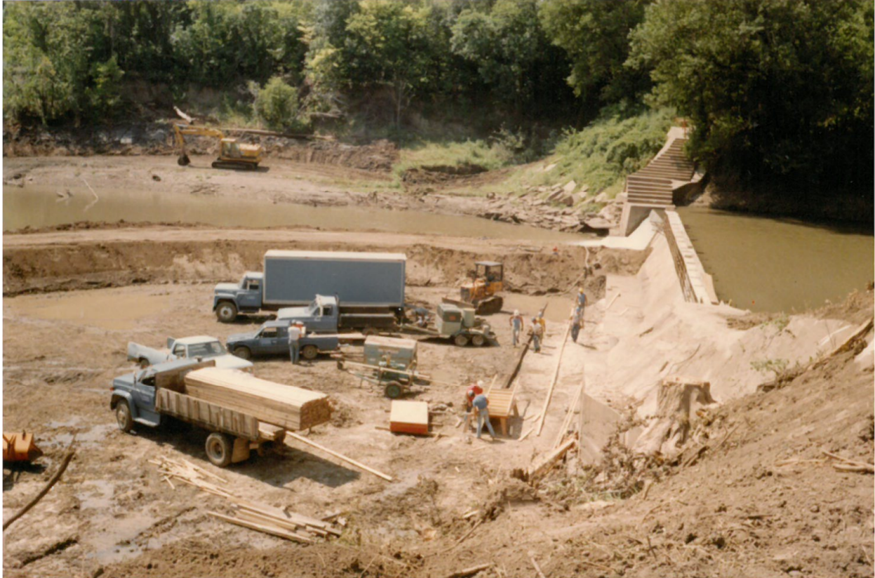
FIGURE 3 - INITIAL DIVERSION OF THE VERDIGRIS RIVER, SEPTEMBER-7TH 1988
