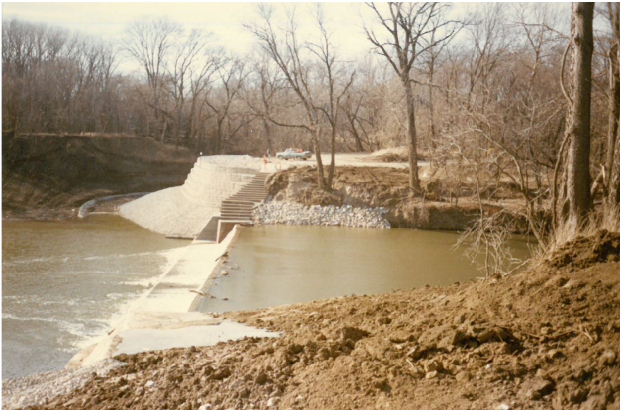
FIGURE 10 - UPSTREAM RIPRAP PLACED, PROJECT COMPLETION, JANUARY 5, 1989
