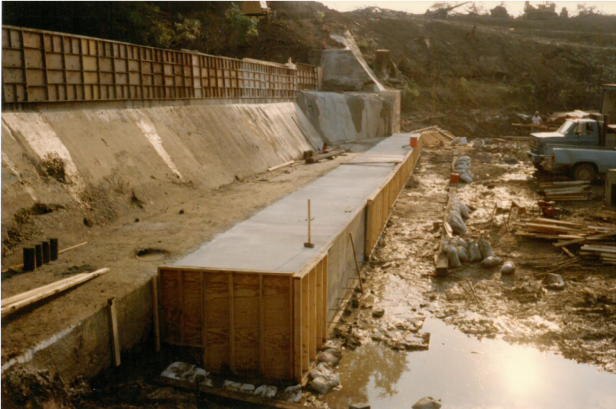
FIGURE 5 - EAST BANK APRON EXTENSION, SEPTEMBER 9, 1988
