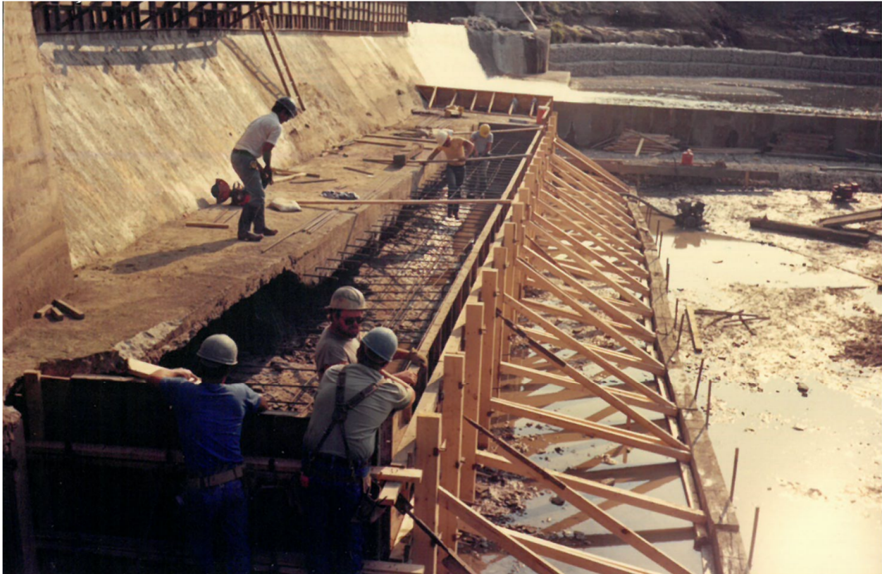
FIGURE 7 - SCOUR REPAIR AND APRON EXTENSION UNDERWAY, SEPTEMBER 13, 1988
