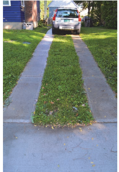
A concrete ribbon driveway in Burlington.
