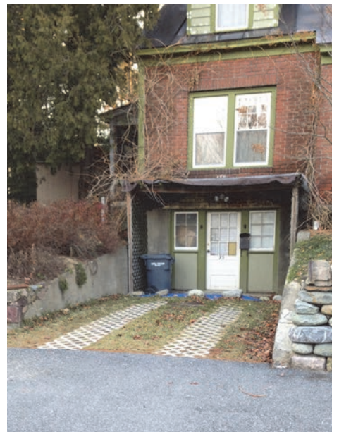
A concrete paver ribbon driveway in Burlington.
