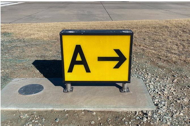
Figure 12: New Taxiway Guidance Sign
