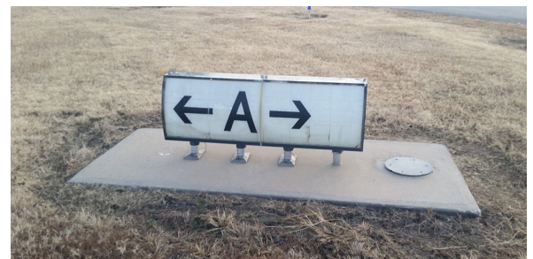
Figure 11: Existing Taxiway Guidance Sign
