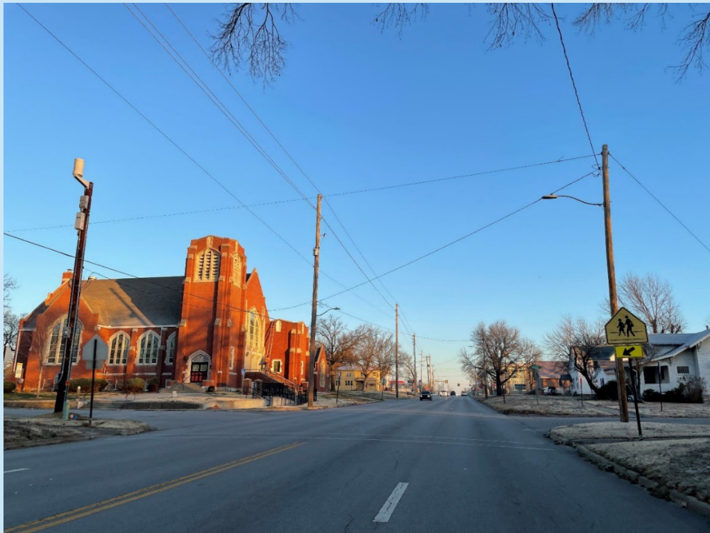
South 10 th Street at West Magnolia Street (Source: FHWA)
