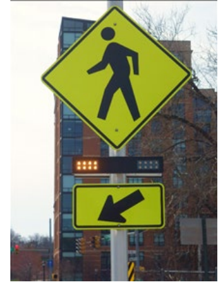
Figure 12. Graphic. Rectangular Rapid Flashing Beacon (RRFB) (Source: FHWA MUTCD)
