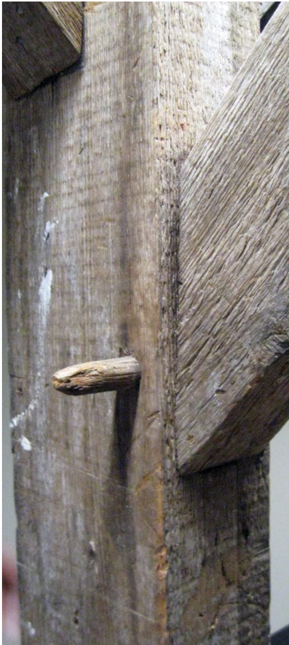
[17] Distinctive examples of traditional construction techniques should be preserved, such as this wooden peg, which is part of the structural system of this late-19th-century warehouse.
