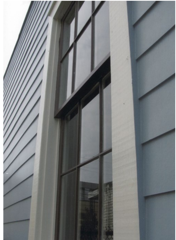
[23] (a) This deteriorated historic wood window was repaired and retained (b) in this rehabilitation project.
