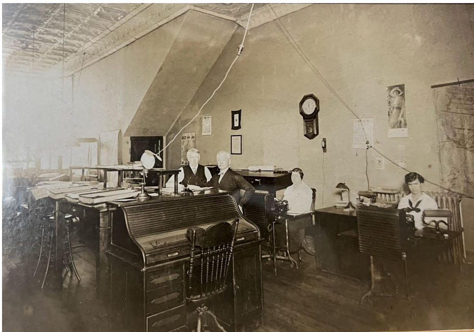
Undated, Interior 1st floor looking Northwest
